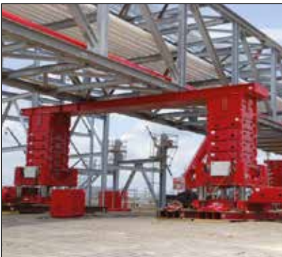
▼ Lifting an oil and gas pipe module.
