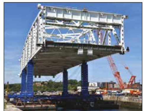
One JS-250 Jack-Up Unit with Barrel Sets installed
