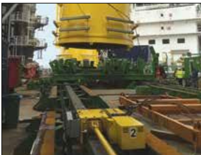
▼ The trolley system speeds up offshore wind transition piece load out: the transition pieces are positioned in the clamping frames and moved along the track.
